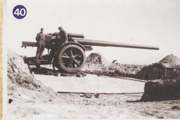
Germans standing by a 15cm army coastal artillery gun in an open concrete emplacement.
