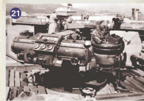
This large German anti-aircraft rangefinder was mounted on the roof of the tower now known as the 'Odeon'.
