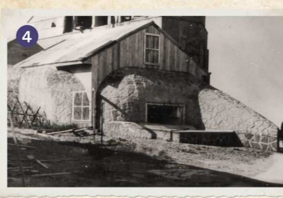
The bunker was camouflaged by the Germans as a house. In the background stands a pre-war stone crusher building since demolished.
